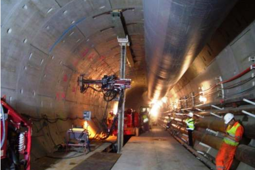
Drill rig mounted on a vertical hydraulic mast
