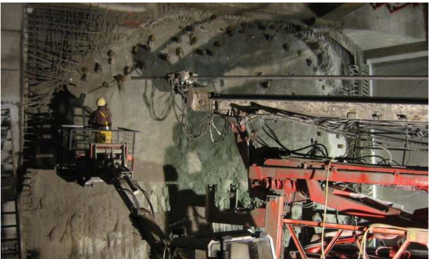
Placement of wooden plug
